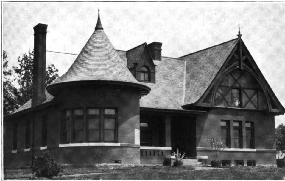
Administration Building STATE FRUIT EXPERIMENT STATION AT MOUNTAIN GROVE
